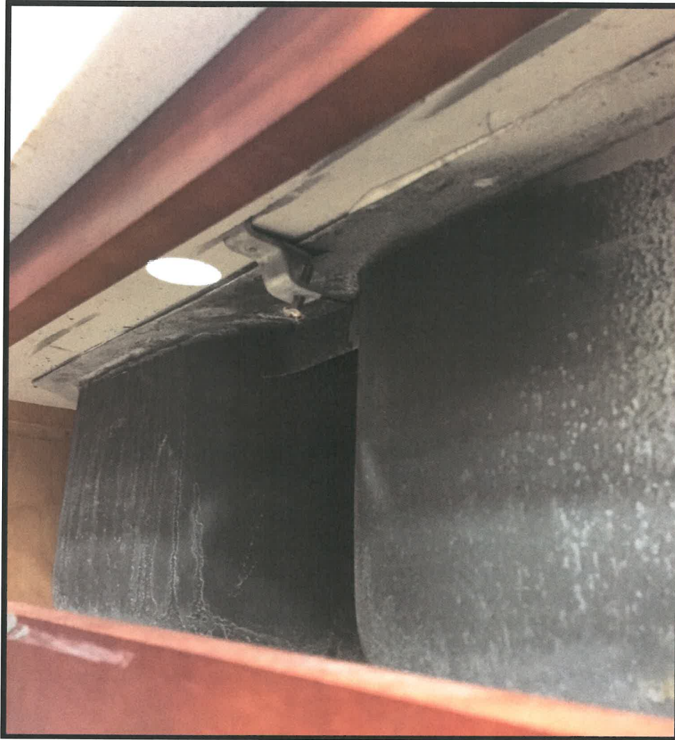
Figure 2: Example of GoClip installed under the countertop
